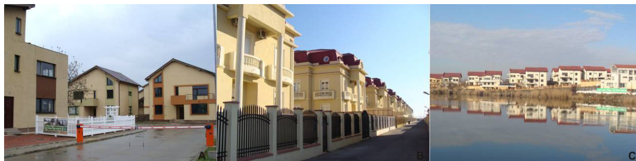
Fig. 8 – Residential development in the Bucharest Metropolitan Area (A – gated community in Corbeanca; B and C – residential projects in Voluntari).
