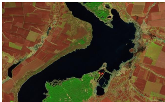
View before the destruction of the dam on March 29, 2022
